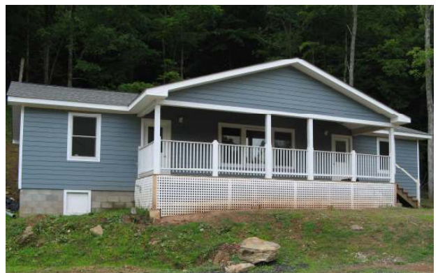
The siding complete and the grass starting to grow!
